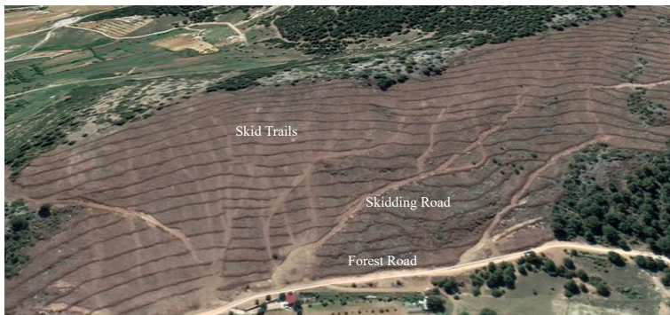
Figure 6. A view of the secondary forest road, skid roads and skid trails together on a stand
