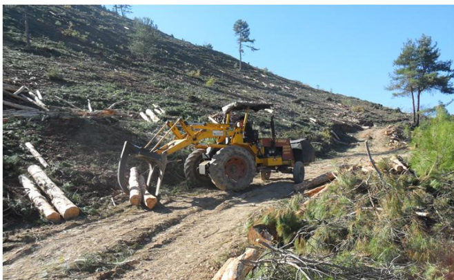
Figure 4. Forwarding with grapple loader on skidding road
