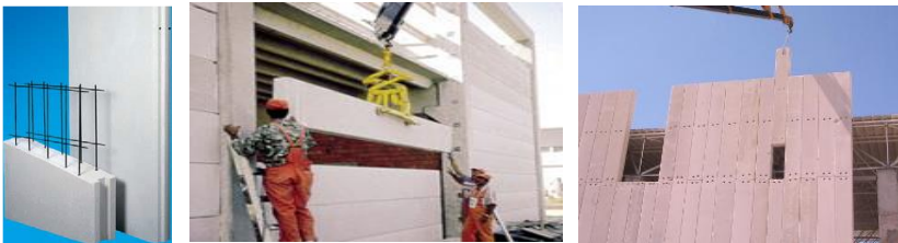
Figure 17. Horizontal and vertical load-bearing wall elements
