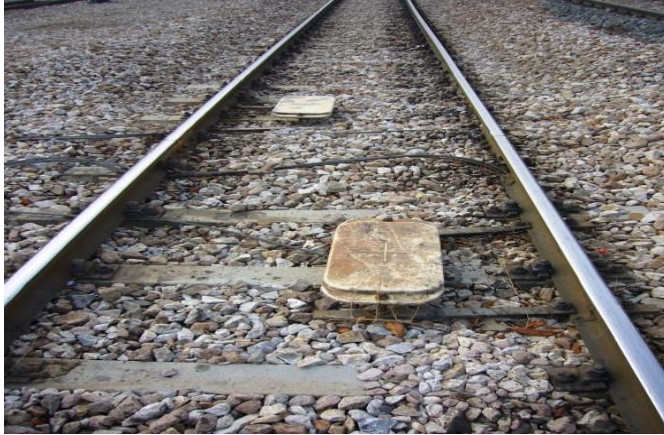
Figure 6: On-Road ATS Magnets
