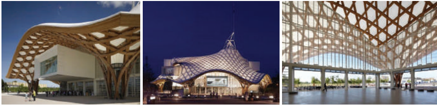
Şekil 6.5. Centre Pompidou-Metz, 2010, Paris, Fransa, Shigeru Ban Architects [37]
